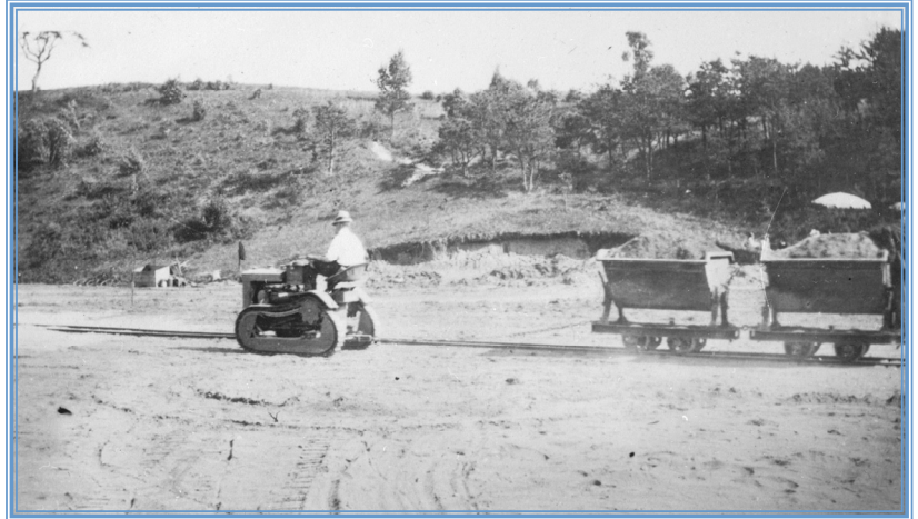
Moving earth by tractor and truck, 1926. Lantern slide 271.
