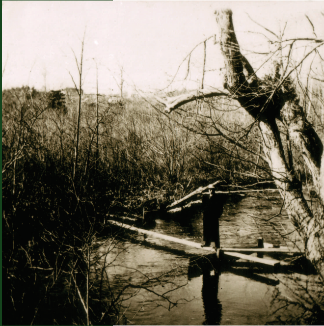
FOOT BRIDGE OVER THE JONES RIVER, BELOW WAPPING ROAD
